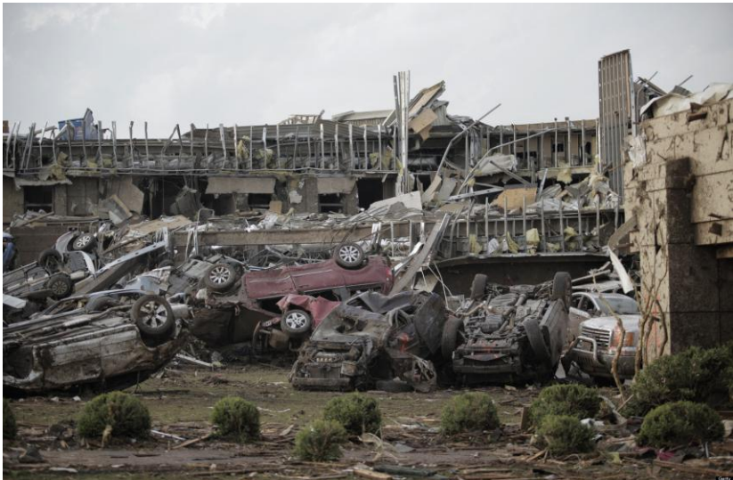
Heavily damaged Moore Medical Center
